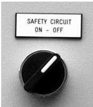
1. Turn "SAFETY CIRCUIT" / "SICHERHEITSKREIS" switch to "OFF".
