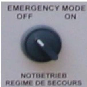
3. Turn the "EMERGENCY MODE" switch to position "OFF".
